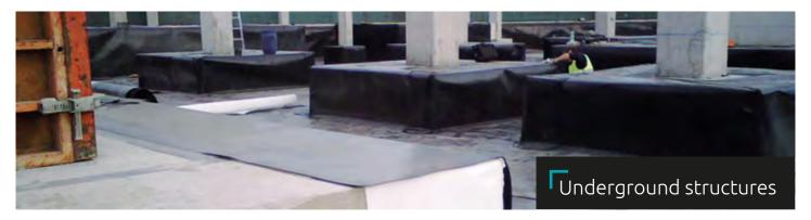
Road and railway tunnels, waterproofing building foundations to prevent damp, and to act as a radon gas barrier.
