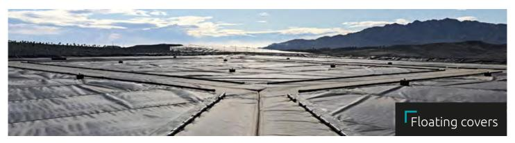
To eliminate evaporation in reservoirs, and deodorise tailings ponds that give off unpleasant-smelling gases.
